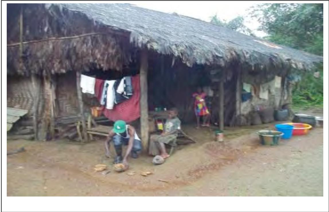
**Figure 17: Typical House unit constructed with piassava fronds and other forest products**
